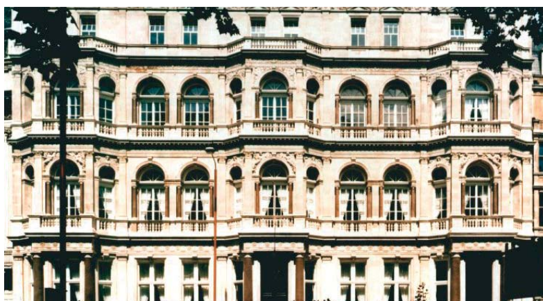
Japanese Embassy Refurbishment London
