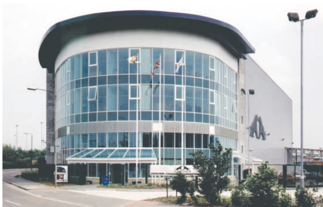
Office & Warehouse Wembley
